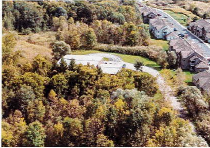
Front Aerial View
