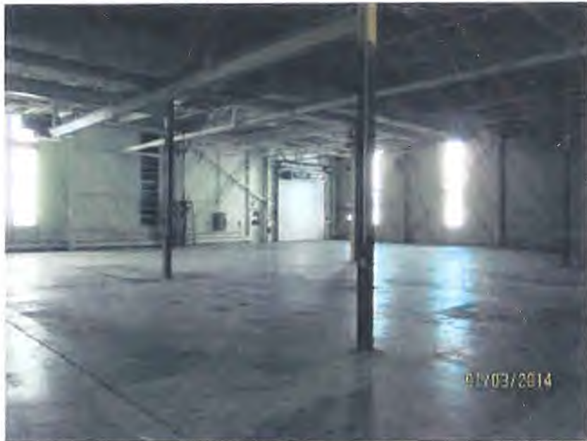
Typical Mfg./Warehouse Area
