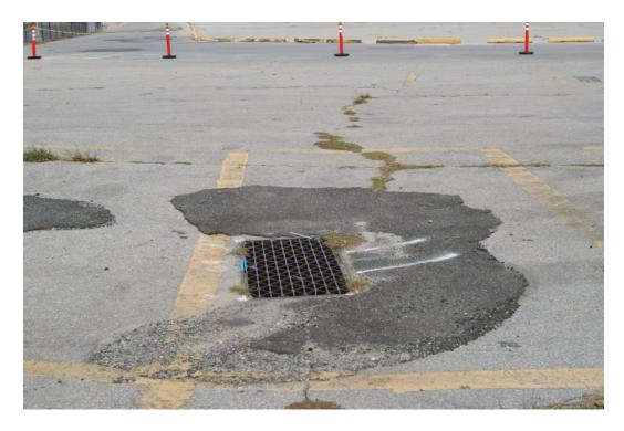
Photos 31E and 38S show the conditions of storm drains on Site A. All observed storm drains were surrounded by excessive pavement cracking and sediment.
