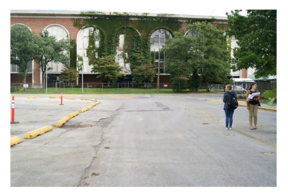
Photos 13S and 19N show cracked and crumbling pavement on Site A.
