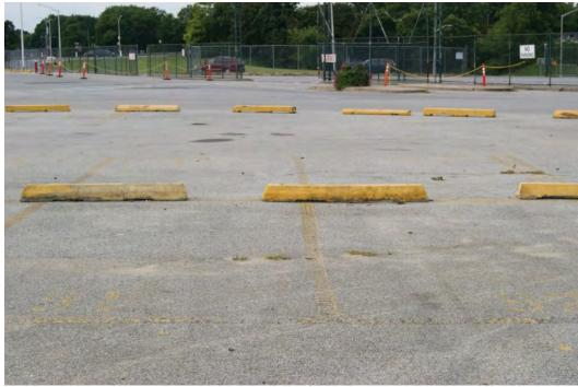
Photos 35N and 8S show the wheel-stops used to define the roadways within the parking lots. These photos also show that the striping in the lot is either missing, needs to be repainted, or does not line up with the wheel-stops.
