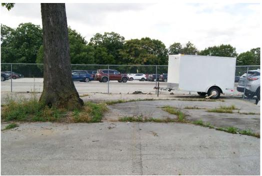
Photos 19S and 67W show trees on both sites that are not protected and interfere with the roadways and parking spaces. Tree roots have led to large cracks and bulges in the pavement. Photo 67W also shows a vehicle trailer with a wheel lock currently stored on Site B.
