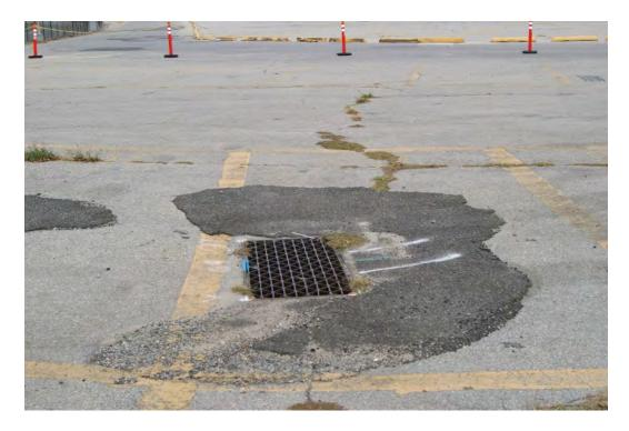
Photos 31E and 38S show the conditions of storm drains on Site A. All observed storm drains were surrounded by excessive pavement cracking and sediment.
