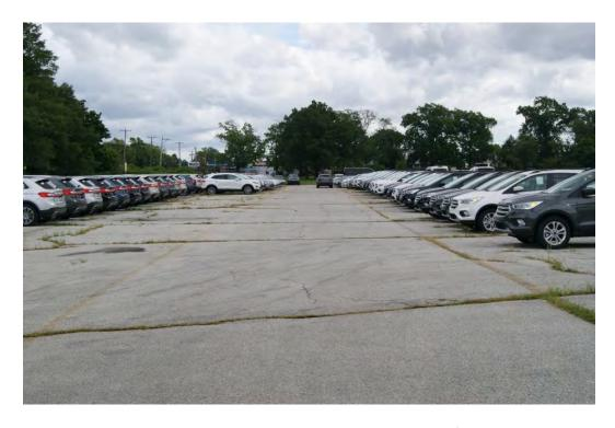
Photo 41E shows cracked pavement on Site B. The cracks on Site B are mostly filled with weeds and vegetation.
