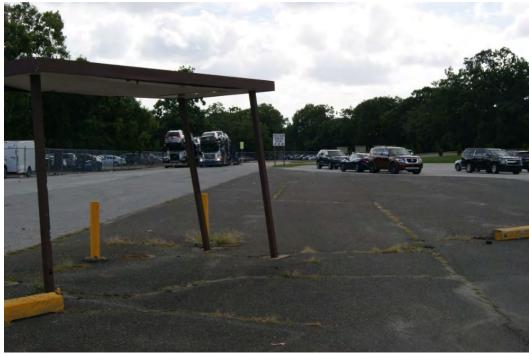
Photos 52N and 65S show the poor conditions of the bus stops on Site B. Bus stops were not observed to be in use during racing days. On one day no buses were used. On the other racing day, a school bus was used to shuttle passengers who flagged the bus down.
