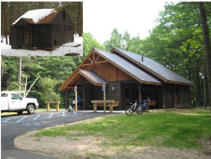
Northampton Campground Comfort Station After
