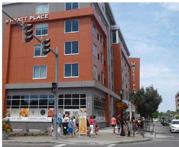
Since 2015, USA Niagara has participated in 7 hotel projects creating approximately 600 new hotel rooms and renovated 357 existing rooms in downtown.
