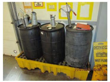
Photograph of waste oil AST in vehicle maintenance building.
