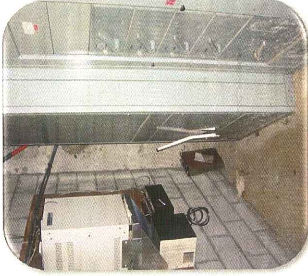
Photo 1 Access to Switchboard's Main Disconnect Switch, in violation of N.E.C. code, is blocked by a control cabinet.
