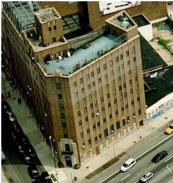
Figure 1: Main Building or West Section
