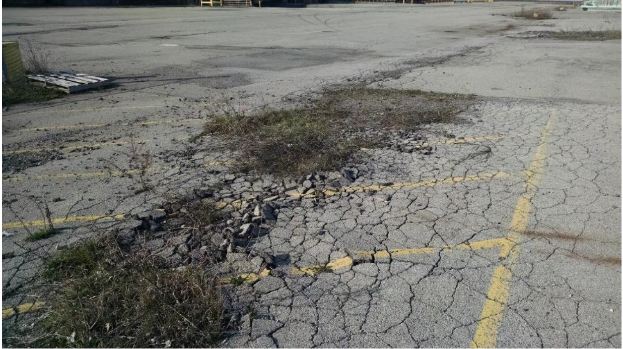
Photo A-13: Terminal A auxiliary parking lot asphalt degradation
