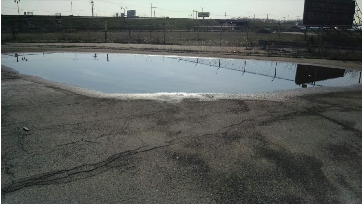
Photo A-17: Terminal A salt storage lot ponding
