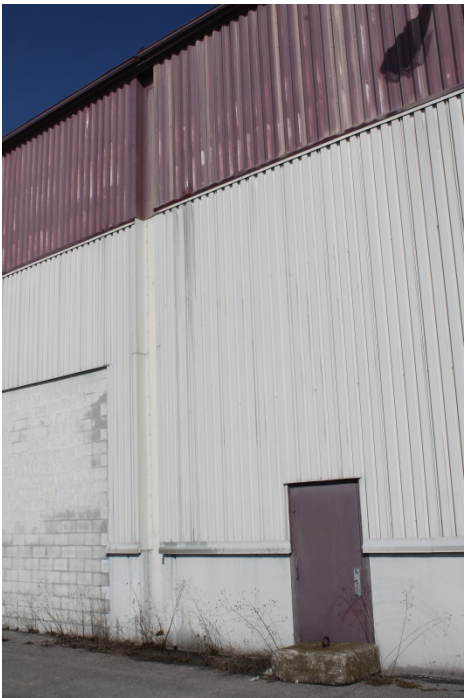
Missing Downspout and Wet Façade
