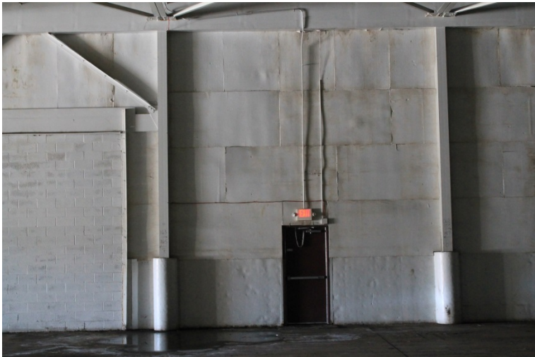
West Wall, Standing Water, Elevated Moisture Readings
